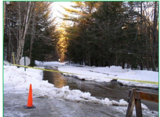
Rowentown Road Flooding Photo Credit: Town of Wentworth
