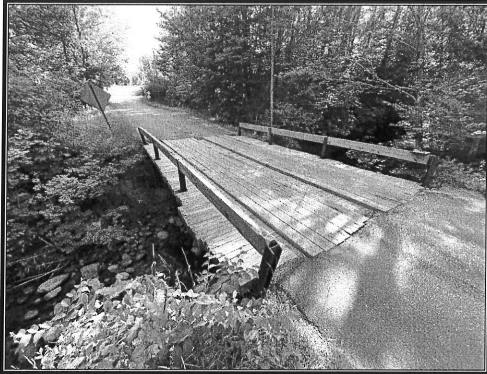
Photo 1: East Side Road bridge.
